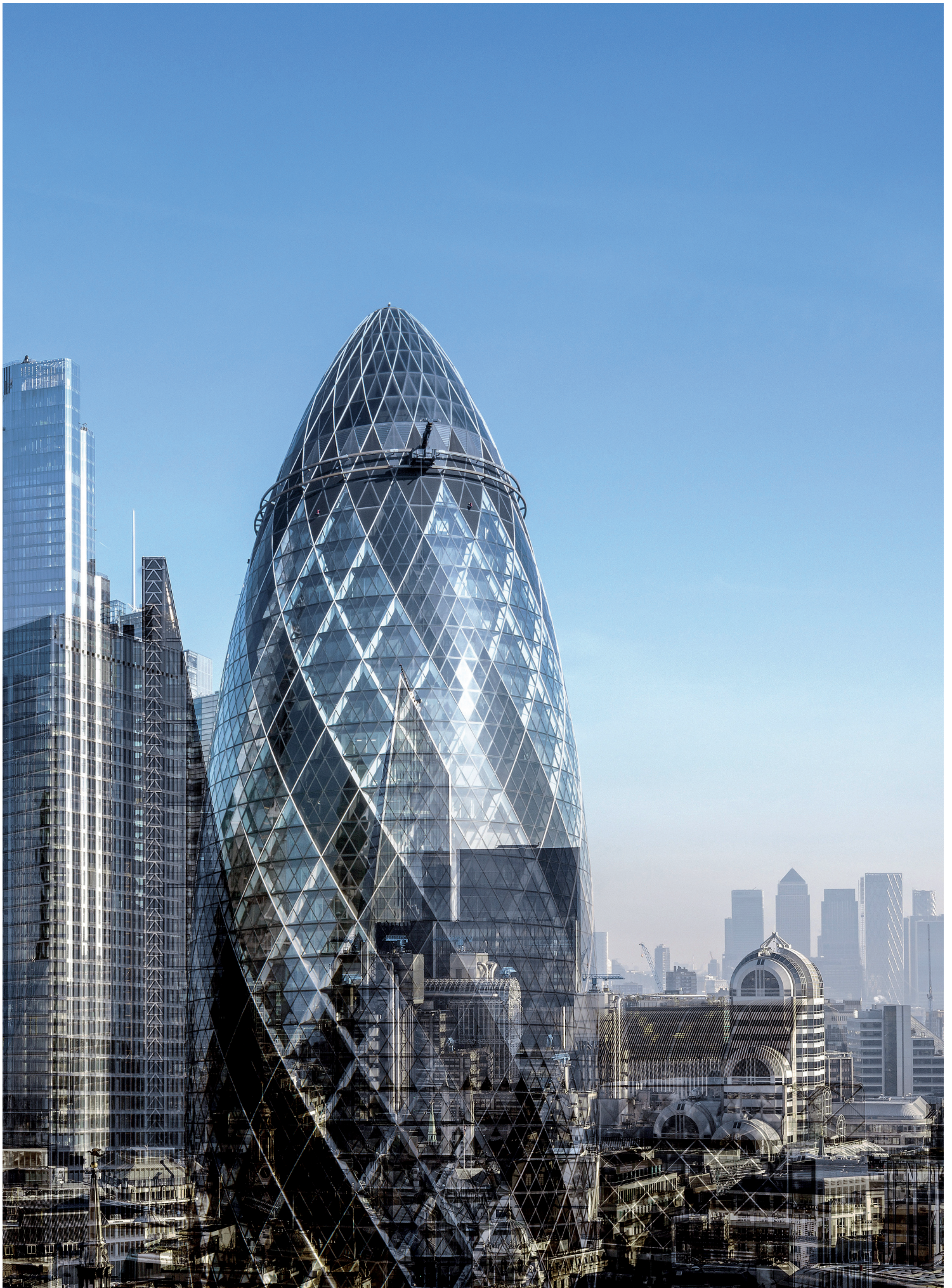
30 St Mary Axe Building, London, UK
