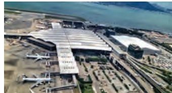
Hong Kong International Airport
