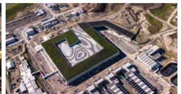
Green Roofing For The Victorian Desalination Plant, Australia
