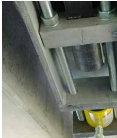
Post-tensioning: a force is applied to create permanent stress in a structure, so that it can withstand load more efficiently or with less total deflection. In conventional post-tensioning, the load is put on steel tendons within the concrete structure, however with the Sika CarboStress® system, the advantages of the Sika CarboDur® CFRP plates and post-tensioning techniques are combined to form a unique active external strengthening solution.
