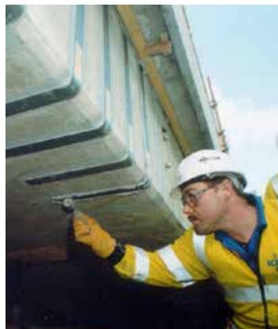
The shear capacity of concrete beams can be increased by the external applied Sika CarboShear L-shaped profiles. Installation is fast and easy, excellent anchorage is assured and no drilling through the top slab is required.
