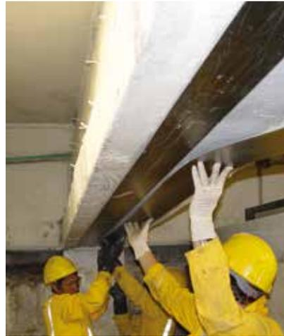
The Sika CarboDur® System is the most widely recognized and established carbon-fiber-reinforced polymer (CFRP) strengthening solution available worldwide. It consists of Sika CarboDur® CFRP plates and rods, together with the structural epoxy resin based adhesives Sikadur®-30 and Sikadur®-30 LP. This simple, tested and well proven, highly durable system has outstanding performance. With the Sika CarboHeater curing times can be accelerated and down time minimized, even at lower temperatures.
