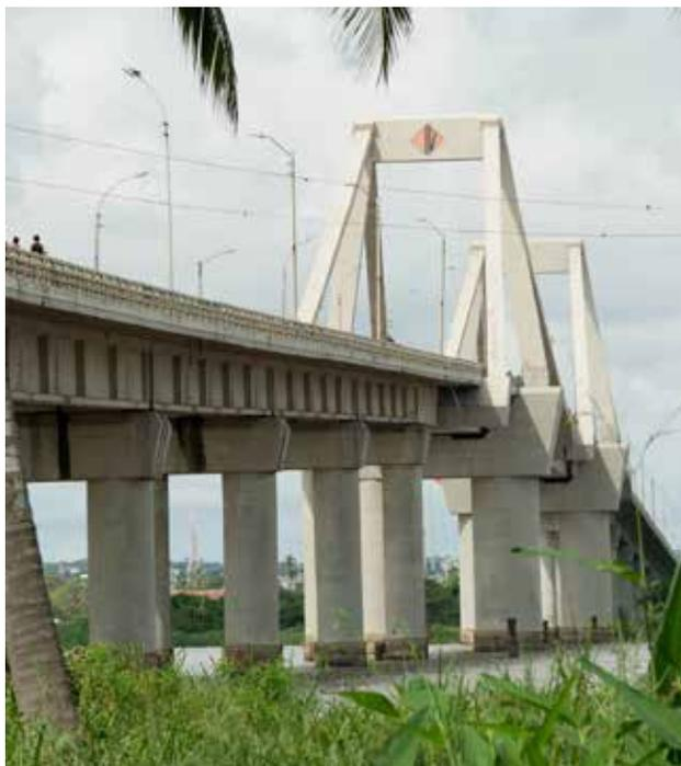
The refurbishment was undertaken in several stages in 2006 and 2008, and it was also decided to strengthen it in 2011. The repair works included removal of weak concrete, cleaning and protection of exposed steel reinforcement, concrete replacement with SikaTop® and EpoCem® systems after crack injection, steel jacketing around the columns, plus overall protection with an impregnating corrosion inhibitor and a protective coating.
